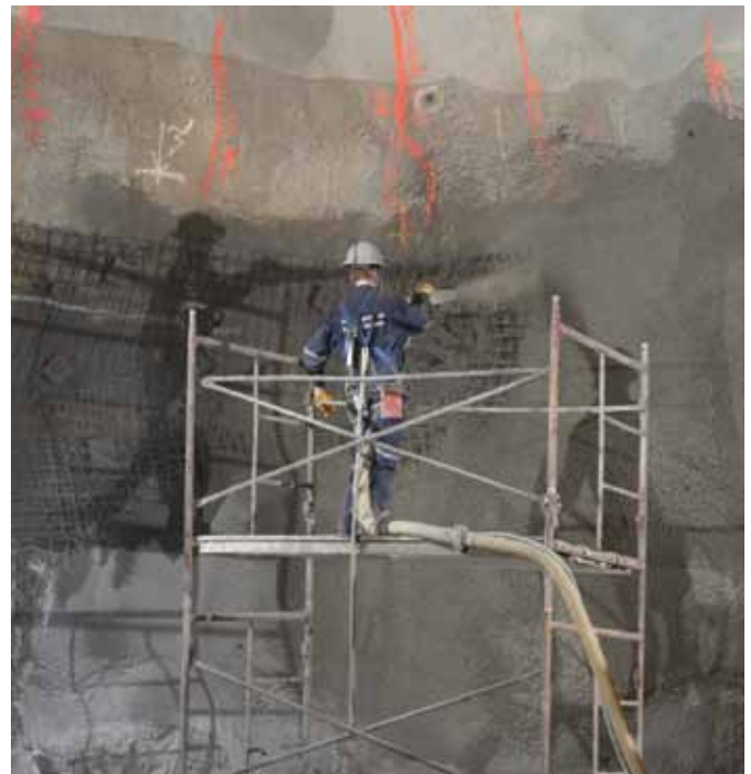
The safest nozzling technique is to straddle the hose and place it between the legs, while maintaining the hose directly behind, to act as a counterweight.
