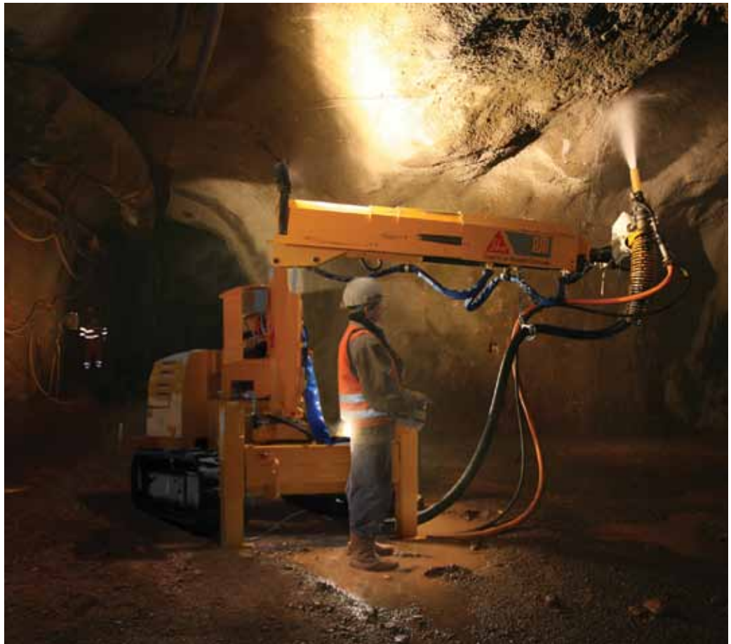
The shotcrete nozzle, in many cases, has been removed from the hands of the nozzleman and placed on a robotic arm.
